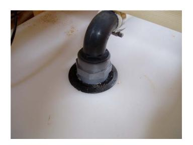
10. Note the special arrangement and different size Uniseal for pump out "dip" tube. This consists of a standard adapter with a collar (which increases the hole diameter required) and a full tank depth, 45° chamfer ended pipe, both permanently attached with solvent weld glue.
