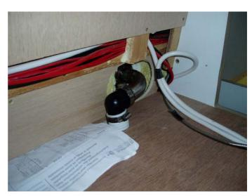
14. If you plan to install a Microvent, product code 02070, this can be installed anywhere in the vent line.
