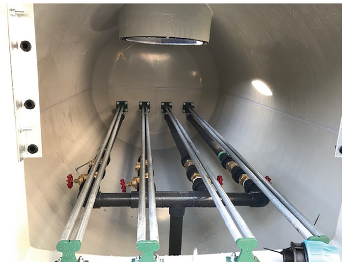
A chamber tailored and designed to specification for Pump Technology, destined for the Marble Arch Tower in Central London.
