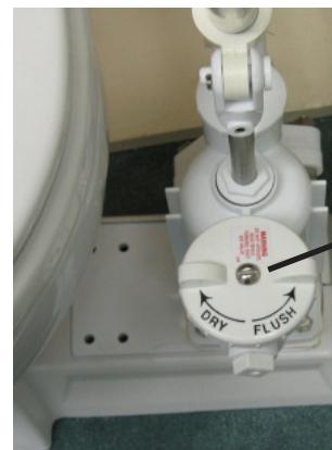
Position for discharge of bowl contents only (no water coming in)
